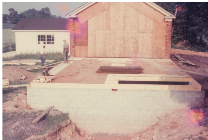
Grange Hall Addition Under Construction
